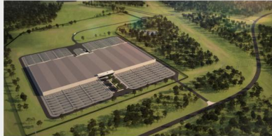
Image: Louisiana Economic Development ( https://www.opportunitylouisiana.gov/news/hut-8-selects-southeast-louisiana-as-site-of-10-billion-artificial-intelligence-data-center )
